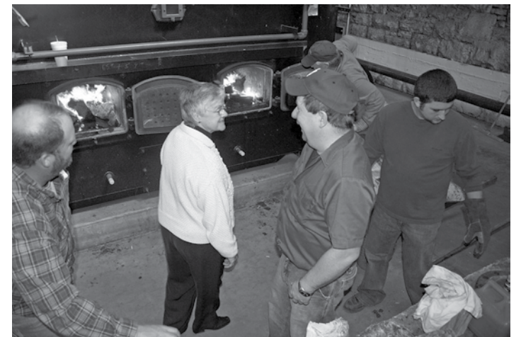
Denise Wilkinson, General Superior for the Sisters of Providence talks with workers in front of the boiler. Photo taken by Cheryl Casselman who is the Marketing Director for the Office of Congregational Advancement for the Sisters of Providence.
